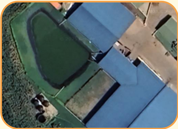
Rainwater Collection System
